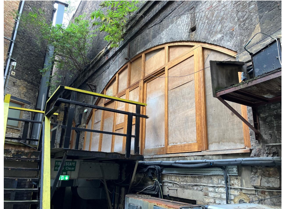
Existing rear archway and escape stairs
